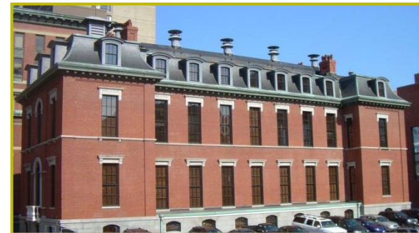
Boston Medical Center BCD Building (Boston, MA)
