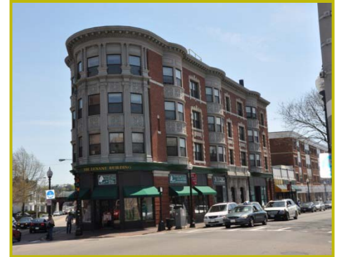
Lenane Building (Boston, MA)
