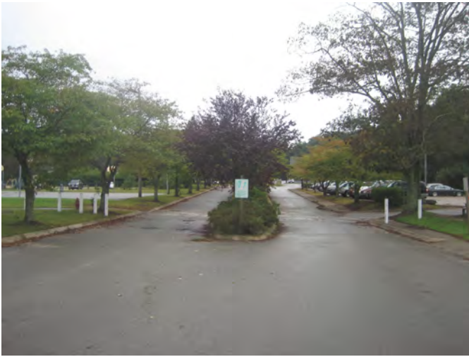
In Wilson Park, a well-landscaped median reduces the expanse of pavement, forcing people driving to slow down.
